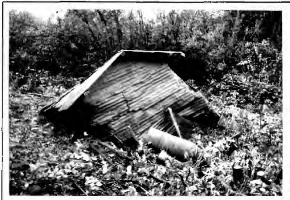
Figure 96. The Anderson Shed ruins, 1993. The view is looking southeast.
